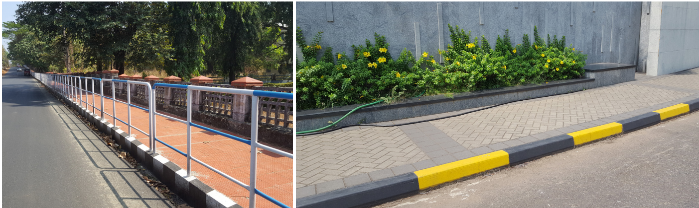
Footpaths with height of no more than 150 mm and colour codes are preferred
